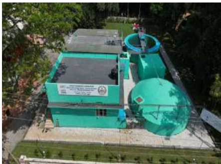
360 KLD STP at General Hospital, Thrissur
