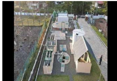
1 MLD CSTP at Padanappalam, Kannur
